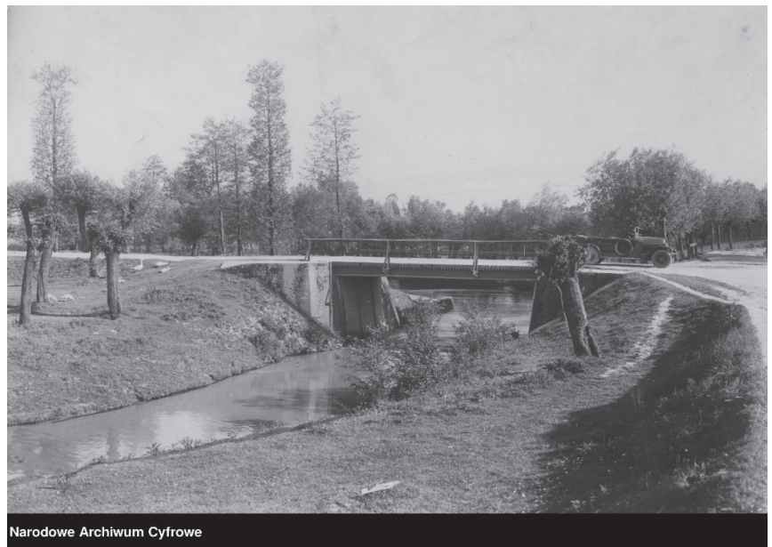
Figure 3. View of a bridge on the Dłubnia, archival photo from 1933. Note the massive concrete abutments that were also used by the weir. From the collection of the Polish National Digital Archives, signature no. 3/1/0/8/3240.
