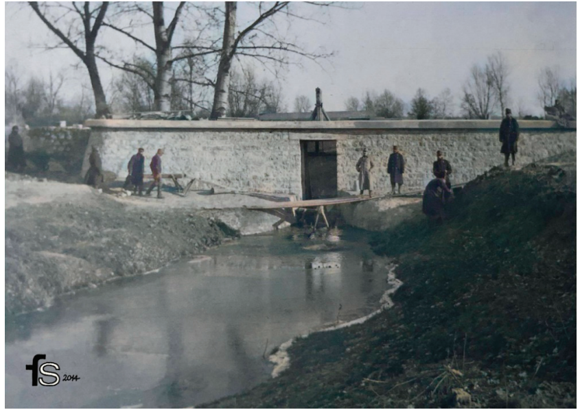
Figure 4. View of the damming wall of the Wilga-Schleufe fortress weir, seen from the side of the inundation area. Archival photograph from 1915. From the author’s collection.
