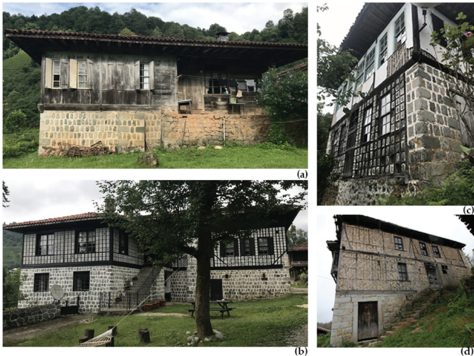
Figure 5. (a) Timber buildings elevated on stone in Hara village; (b) stone-infilled building in Çağlayan village; and (c) mixed construction on a building in Hara village. The stone and stone-infilled technique on the ground floor and the plastered façade of the first floor is an example of the çakatura technique. Source: Photograph by the first author taken in July 2019. (d) Amulet-filled building in the district of Pazar in Rize. Source: https://karadeniz.gov.tr//konut-ahmet-sakir-efendi-konagi/#prettyPhoto (accessed on 8 February 2022).
