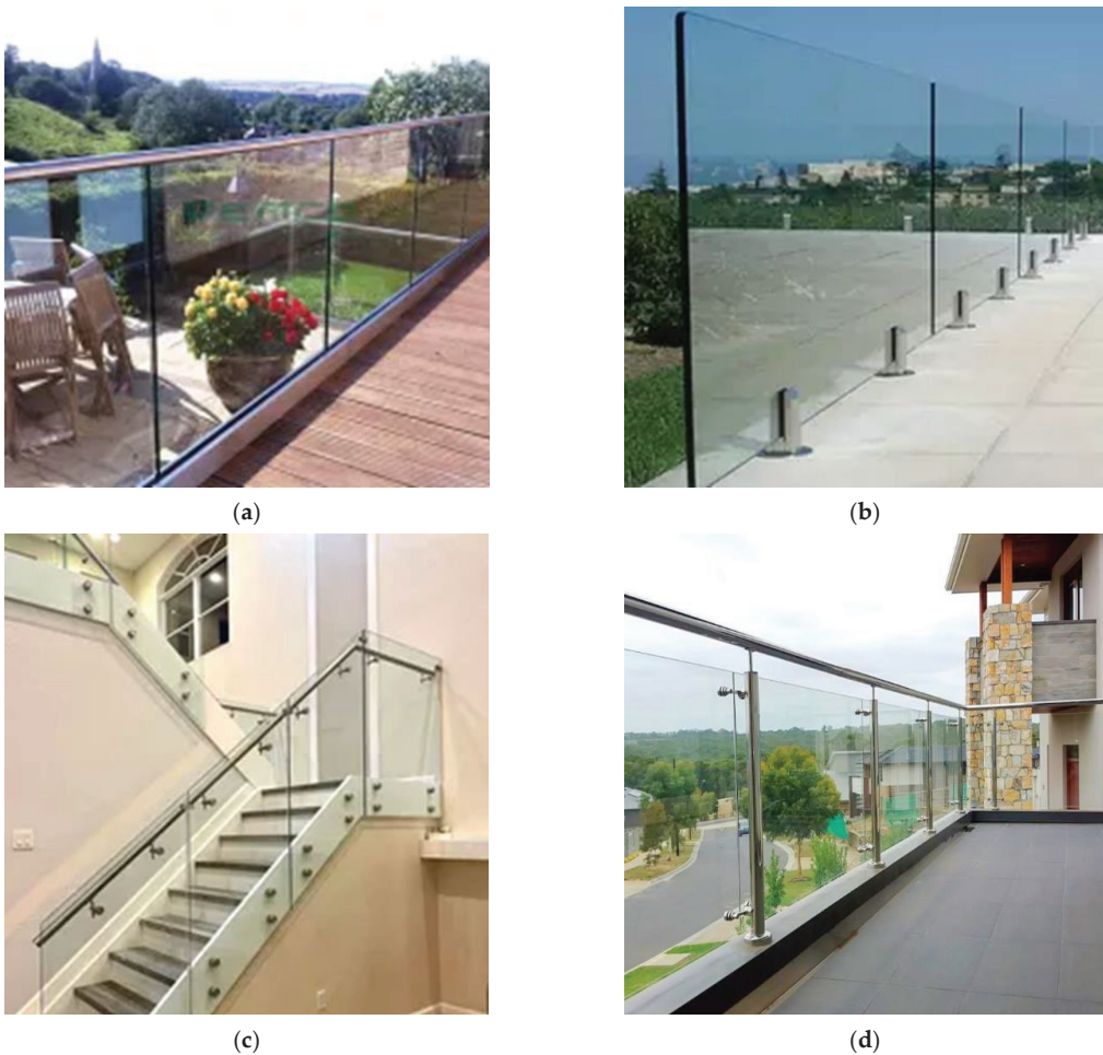
Figure 1. Examples of glass balustrades characterized by various restraint conditions: (a) linear restraint at the base; (b) point-fixing at the base; (c) top-bottom point-fixings; (d) lateral point-fixing. Solutions (a,b) do not require glass drilling; (c,d) are characterized by the presence of glass holes.
