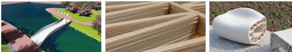
Figure 1. First 3D-printed bridge in China, Shanghai (left); 3D printing infill pattern (middle); 3D-printed cross section (right) [28].
