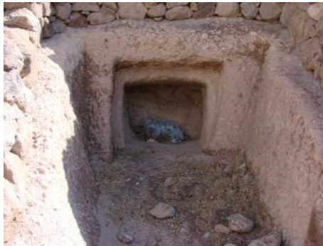
Figure 20. An unfinished kicheh in Meymand shows that the doorways should be completed before moving to other elements.
