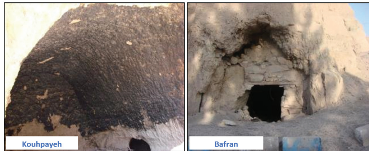
Figure 9. Arched excavation in the form of barrel arch in Kouhpayeh of Kerman and Bafran of Naein.
