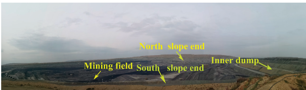
Figure 2. High slopes of Shengli #1 open-pit mine.
