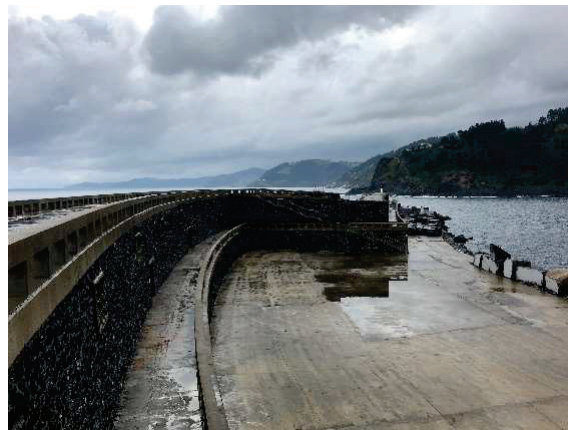
Figure 9. Mutriku OWC plant.
