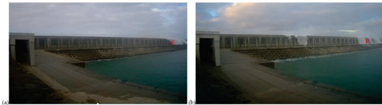
Figure 8. Aspect of overtopping event during (a) storm c and (b) storm d (monitoring section represented by a red line).
