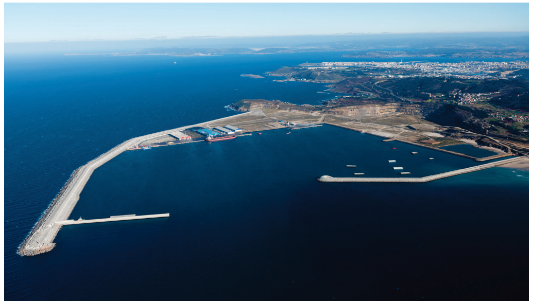
Figure 1. Aerial view of the outer port of Punta Langosteira, A Coruña, Spain.
