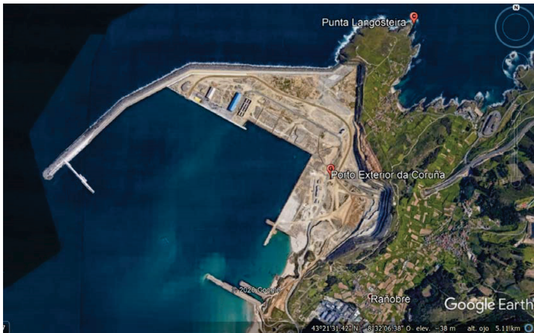
Figure 1. Outer Port of A Coruña “Langosteira” (Google Earth).
