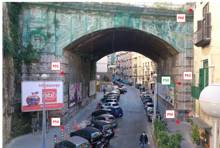
Figure 6. View of the north facade with markers locations. GCPs are represented in red while CP is represented in green.
