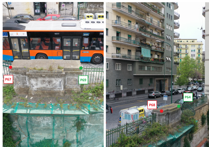
Figure 7. View of the north side part of the extrados with markers locations. The left image refers to the left part of the extrados while the right image to the right part. GCPs are represented in red while CPs are represented in green.
