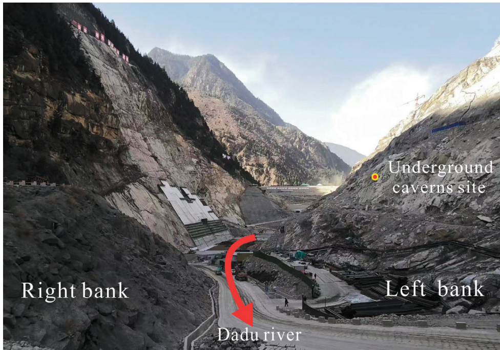
Figure 3. Dam site of Shuangjiangkou Hydropower Station.
