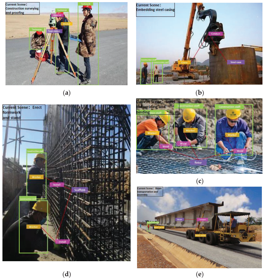
Figure 6. Partial results of the bridge key construction scene identification method on the test set. (The sources of the identifiable images in Figure 5 are shown in the Supplementary Materials.)
