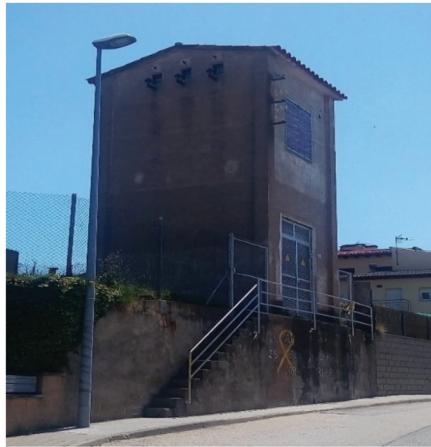
Figure 5. A picture of SS-B where the PED and the batteries were installed.
