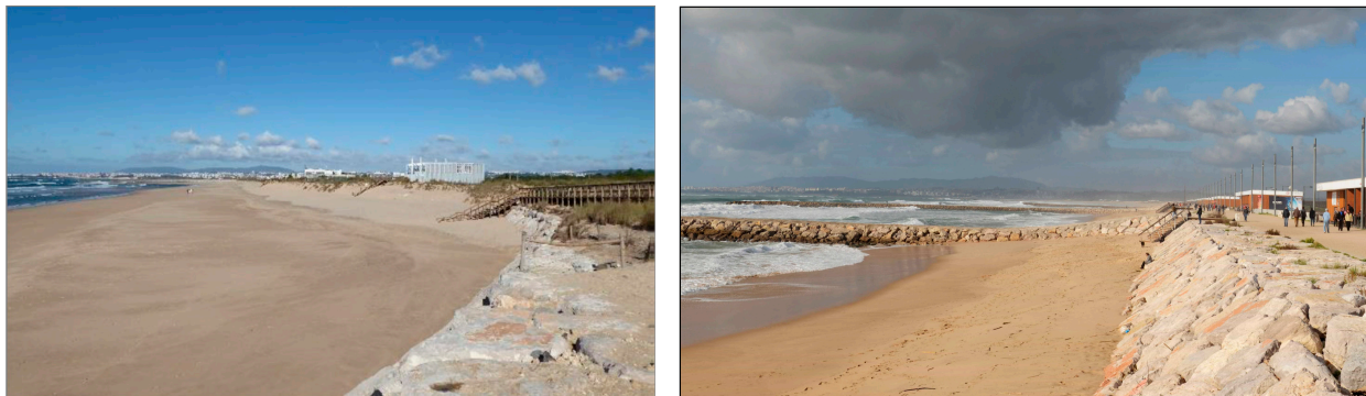
Figure 2. Images of Costa da Caparica beaches: Praia de São João da Caparica (left), and central urban beach, confined by groynes and an inland revetment (right).
