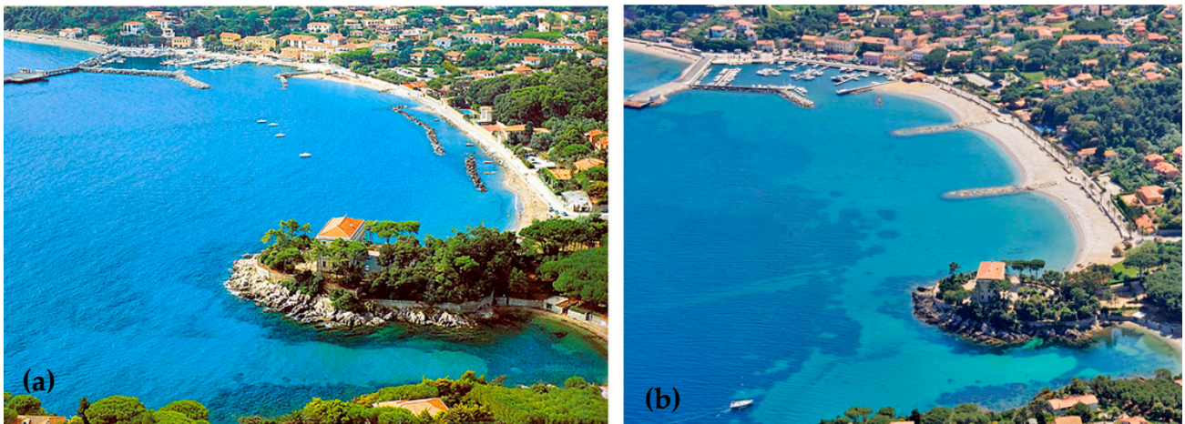
Figure 13. The beach at Cavo before (a) and after (b) the works (Courtesy Elbaworld).
