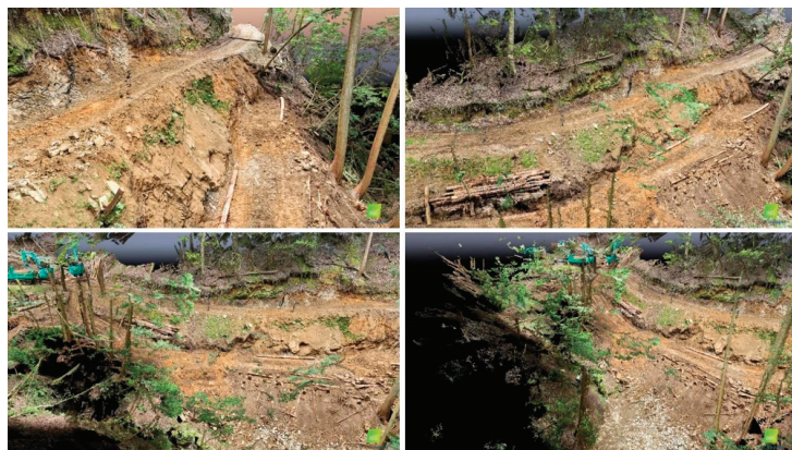
Figure 2. A 3D model generated by SfM analysis during the repair work.
