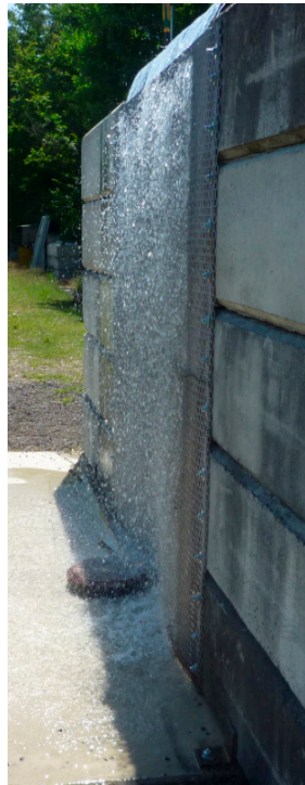
Figure 8. First grid equipped with a pool fountain.
