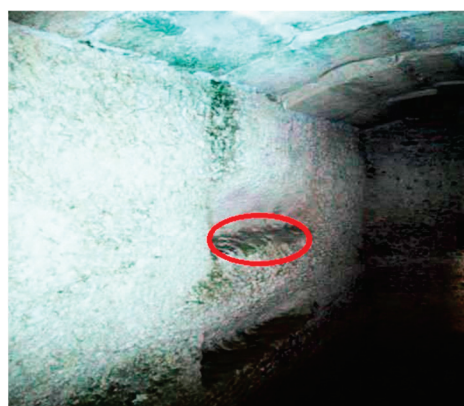
Figure 12. Study area with bio-patina in the hypogeum of San Pietro Barisano church. During the cleaning test, the microclimatic conditions of the wall surface portion sampled were locally ranging between 89–92% humidity and 11–16 °C temperature.
