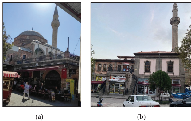
Figure 2. (a) İzmir Başdurak Mosque is located at the lower level of the large-scale commercial unit (b) Afyon Yoncaaltı Mosque, where small-scale commercial units are located at the lower level.
