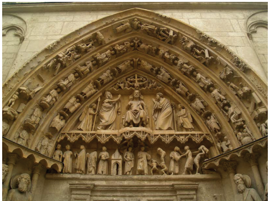
Figure 2. Tympanum of the Coronaria Portico, c. 1245–1257. North façade of the Burgos Cathedral.
