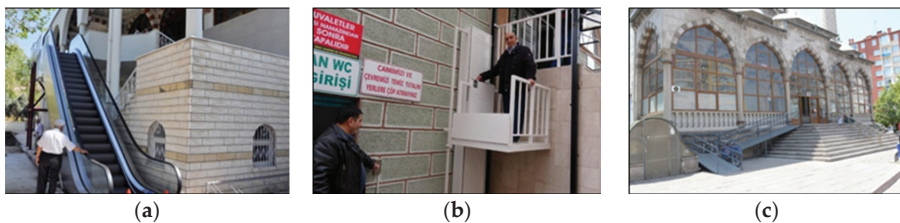
Figure 20. (a) Meltem Mosque, escalator solution; (b) Green Mosque, elevator solution; (c) Melikgazi Mosque, ramp solution.
