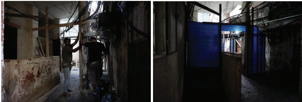
Mode 2: (L) Constructing the UN shelter room, (R) Shelter room installation in blue (the official UN color) intersecting with the existing spatial fabric causing the blue shelter to be interrupted on all four sides.
