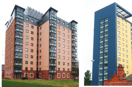
Figure 4. City West Housing Trust high-rise blocks after works.
