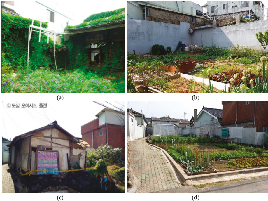
Figure 1. (a) Site A before vacant house was demolished (source: Daegu city hall); (b) Site A after vacant house was demolished (photo: J. Lee, 2 April 2016); (c) Site B before vacant house was demolished (photo: Oasis Plan); (d) Site B after vacant house was demolished (photo: J. Lee, 23 May 2016).
