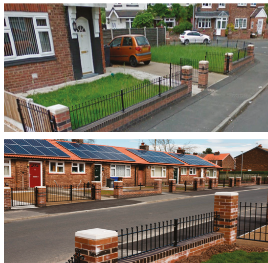
Figure 6. City West Housing Trust “environmental” scheme after works.
