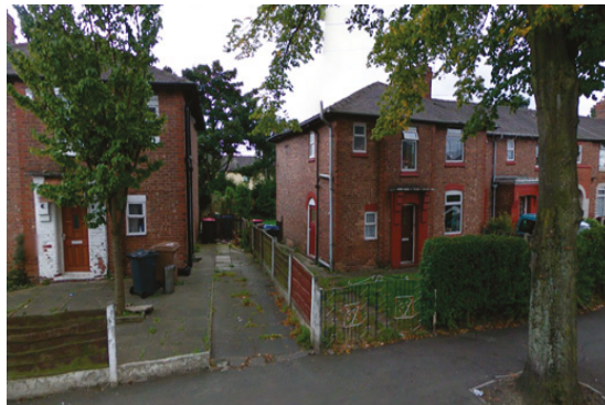
Figure 5. City West Housing Trust “environmental” scheme before works.
