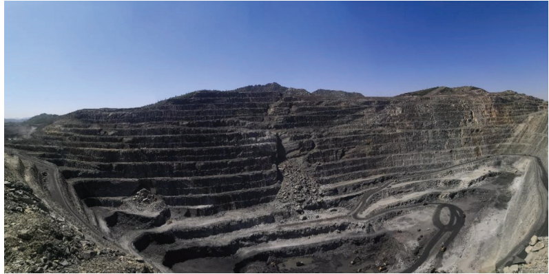
Figure 1. Open-pit mine slope from the radar perspective.
