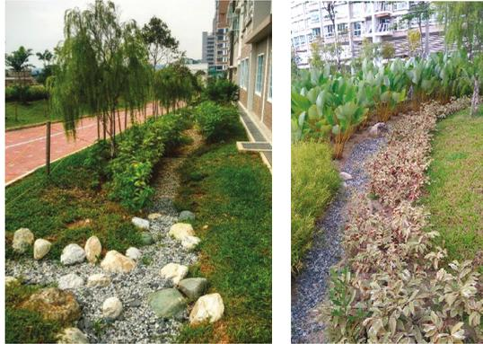
Figure 5. Photos of vegetated swales in Waterway Ridges.
