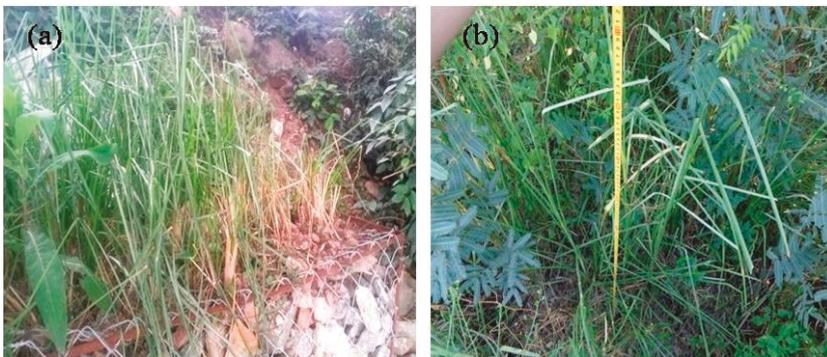
**Figure 8.** Vetiver growth on: (a) gabion; and (b) riprap revetments (photos were taken on 23 October 2016).
