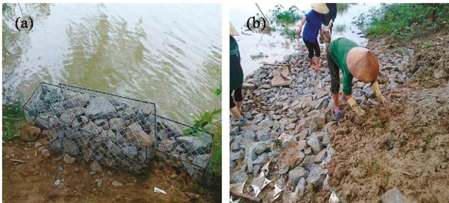
**Figure 4.** Experimental site: (a) gabion; and (b) riprap revetments (photos were taken on 19 November 2015).
