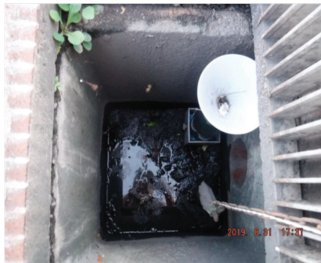
Figure 2. Inside the street stormwater inlet.
