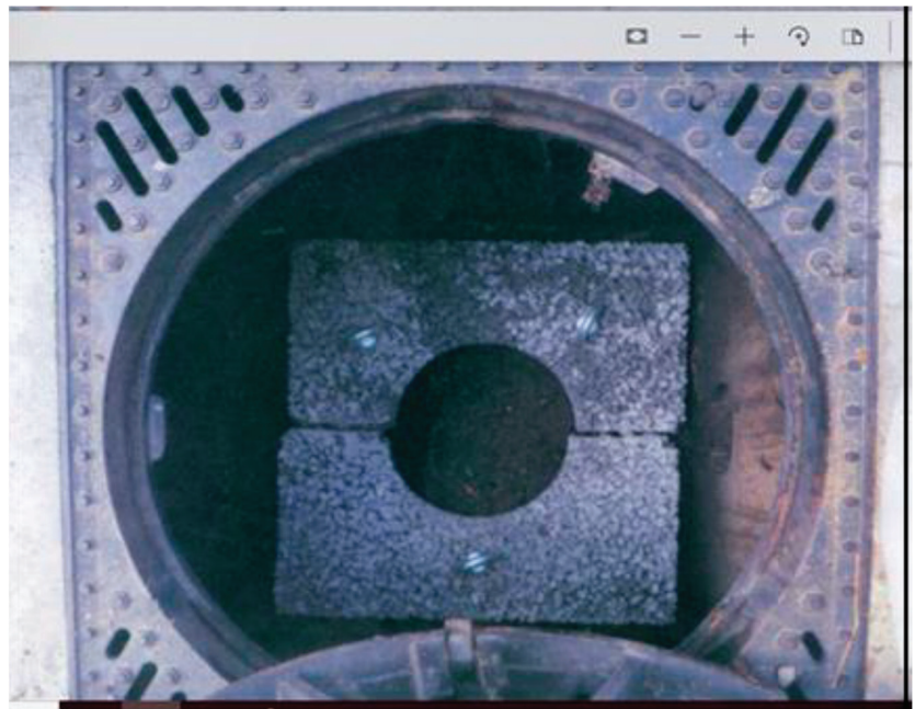
Figure 9. Porous concrete plate at the bottom of the street stormwater inlet.
