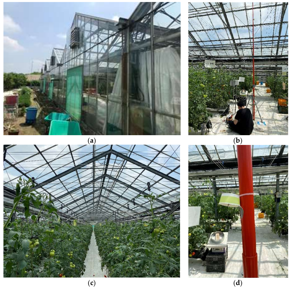
Figure 4. Experimental greenhouse located in Moga-myeon, Icheon-si, Gyeonggi-do Province (37° 18'N, 127° 48'E) and field experiment (a) External view of the experimental greenhouse, (b) Sensor installation for measuring vertical air temperature, (c) Internal view of the experimental greenhouse and (d) Sensor installation to avoid direct radiation.
