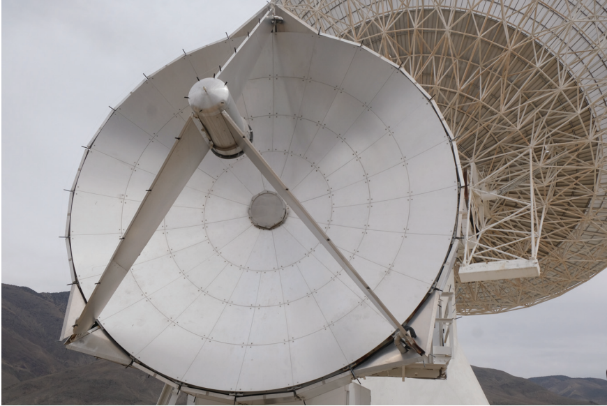
Figure 14. Photograph showing the condition of the BIMA antenna dish surface (from March 2022).
