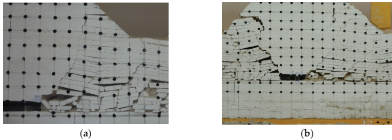
Figure 6. Overburden damage of roadway. (a) Cracks develop to the surface. (b) Roadway damaged by extrusion.
