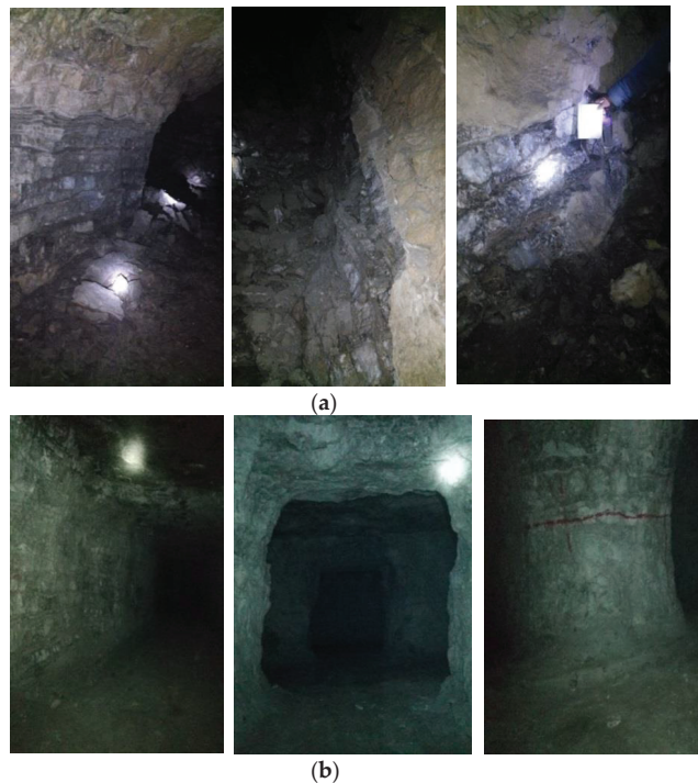
Figure 6. Pictures of gypsum rock pillars in different years. (a) Formed in 1996 and (b) formed in 2017.
