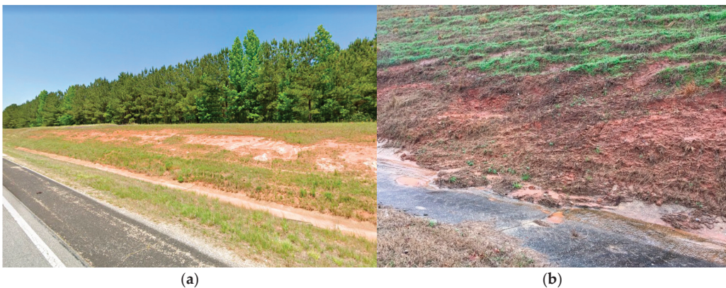
Figure 1. Eroded slopes along (a) US-280 near Waverly, Alabama (photo from Google StreetView) and (b) Alabama Highway 69 near Tuscaloosa, Alabama (photo provided by Jacob Hodnett, ALDOT).
