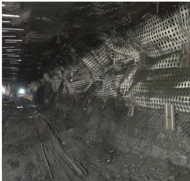
Figure 26. Effect picture of on-site support.
