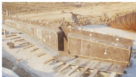
(c) Formwork assembling
