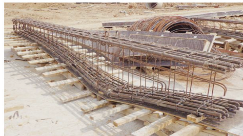
(a) Rebar binding
