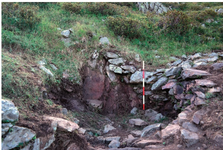
Figure 16. Fusine (SONDRIO), Val Cervia. roasting furnace to the south of the mine. Detail of the combustion chamber which has partly collapsed and been filled with debris.
