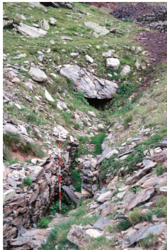
Figure 8. Piateda (SONDRIO), mining complex of Venina. View of the underground entrance to the mine with the access corridor outside (image by the Author).
