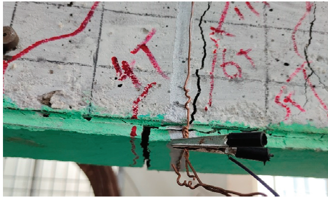
Figure 7. Failure modes of the smart mortar layer.
