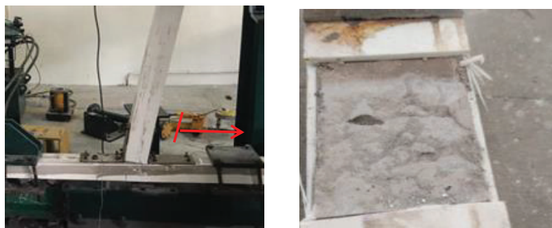
Figure 8. Failure pattern of beam-columns manufactured from GFRP infilled with and without HVFA-ECC.
