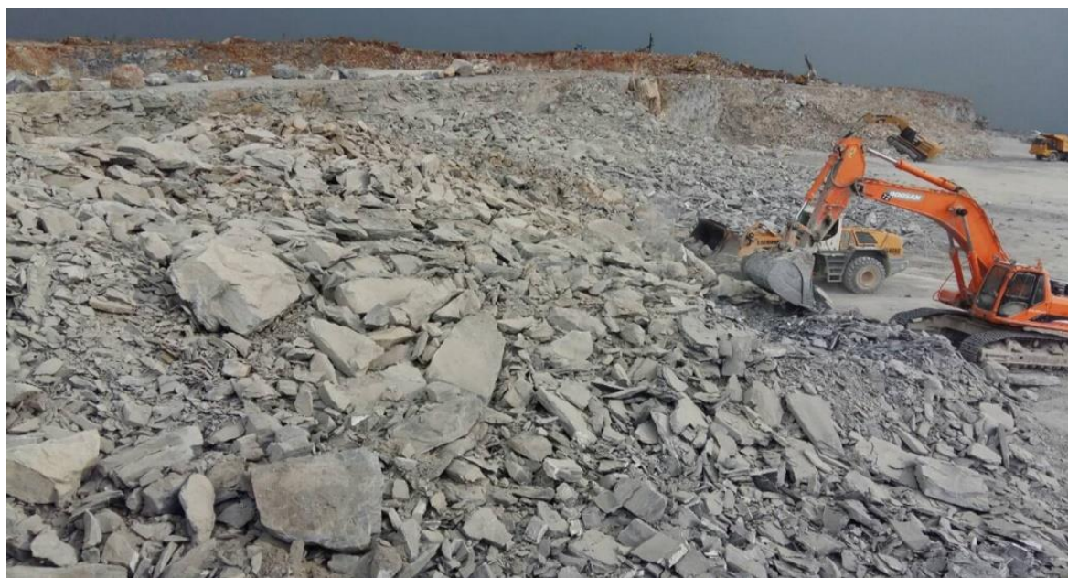
Figure 6. Blasted stone muck pile at quarry face.
