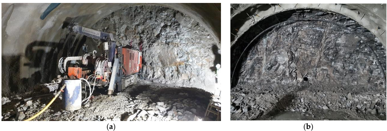
Figure 2. Images of field application of the LLB machine and a tunnel face with completed drilling. (a) Field application of the LLB machine; (b) tunnel face with completed drilling.
