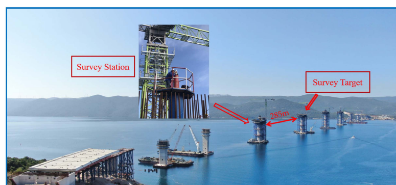
Figure 2. The offshore survey layout of the Peljesac Bridge.
