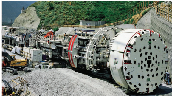
Figure 4. The earth pressure balance shield TBM used.
