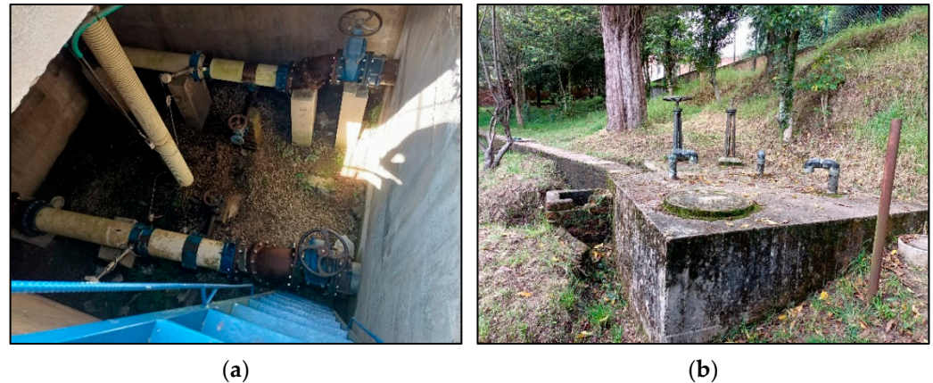
Figure 5. Record of field inspections. (a) Piping and valves; (b) pressure-bursting chamber 4.
