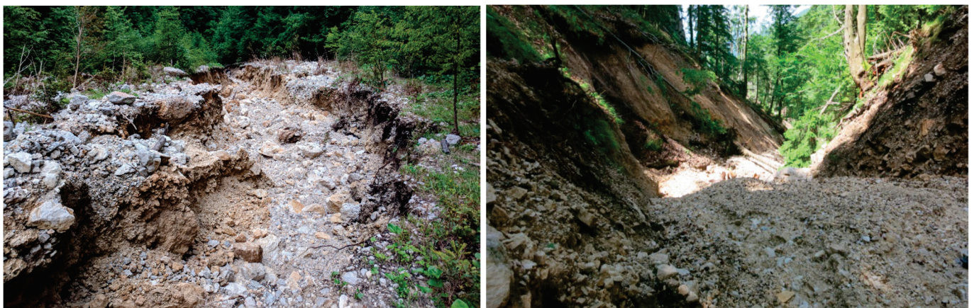
Figure 2. Two photos of the situation in the Brezovški graben and Lukenjski graben torrents, respectively. The channel width is between 1–2 m to several meters.
