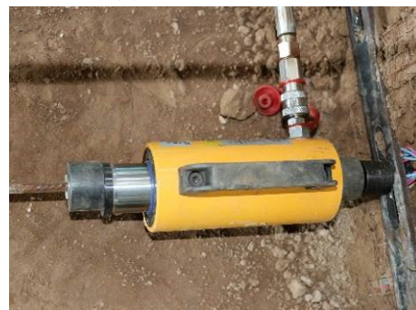
(c) Tension anchors
