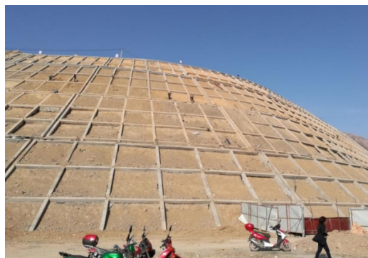
Figure 2. Filled-slope reinforced by a frame with prestressed anchor-plates.
