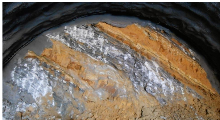
Figure 5. Calcareous sandstone facies with isolated intercalations of marl material, recognized in the advance of Axis 1.
