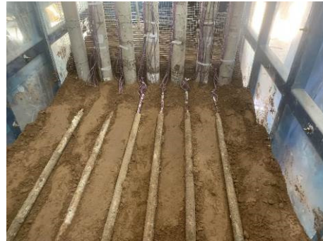
(a) Anchor installation
