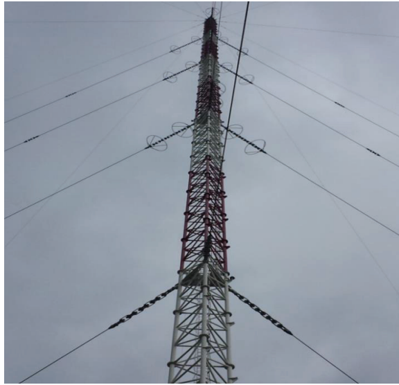
Figure 2. Single umbrella antenna of Changhe II.
