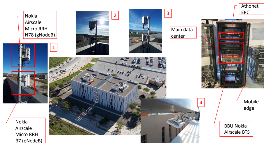
Figure 3. 5G NR NSA deployment at UMA campus. The operation band is also reported for the Radio Remote Heads (RRHs) forming gNBs/eNBs, numbered from (1) to (4).
