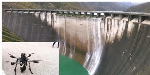
**Figure 2.** Ridracoli dam while overflowing. Small panel: HIGHONE 4HSEPRO quadrotor mounting a gimbal system and a SONY Alpha 7R while at rest.
