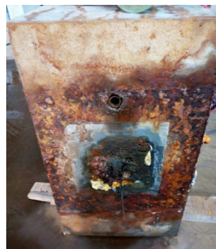
Figure 3. Corrosion fracture at end anchorage part of steel strands in test members.
