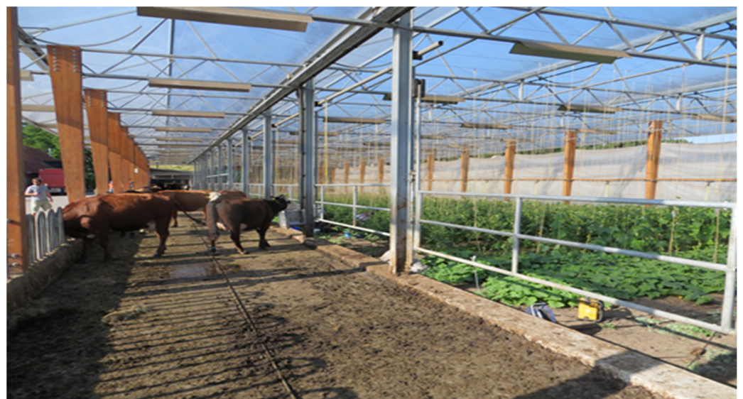
Figure 6. Utilizing a compost bedded-pack barn for growing horticultural products. Source: Farm Veld & Beek, Doorwerth, the Netherlands.
