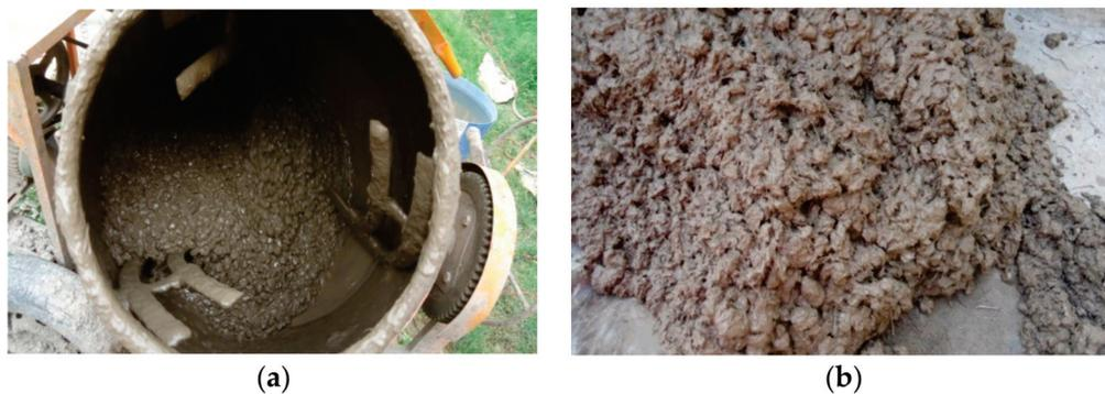
Figure 2. (a) The mixing of ingredients in a mechanical mixer. (b) The freshly prepared SF-reinforced GPC mixture.
