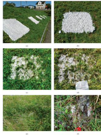
Figure 3. Photographs of the installed prototypes, (a) installed prototype 1–6, (b) day of installation, (c) after 11 weeks, (d) after 22 weeks, (e) after 35 weeks (f) close-up view after 35 weeks.
