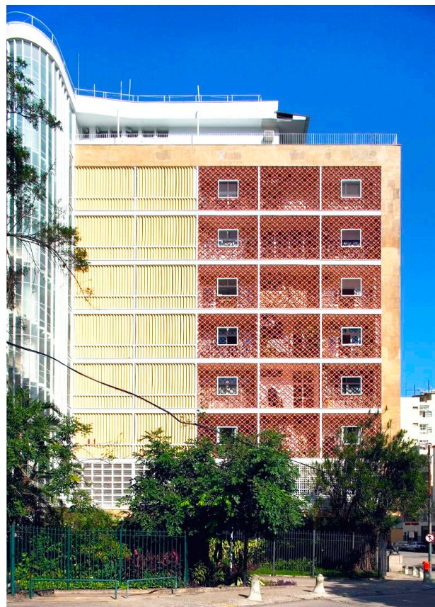
Figure 2. Nova Cintra building north façade, with the façade three main shading systems: the ceramic cobogó with window, the ceramic cobogó without window and the concrete brise-soleil. There are two other shading systems, the lattices and the shutters, both from wood, applied only in the building’s first floor. Photo credits, the authors.
