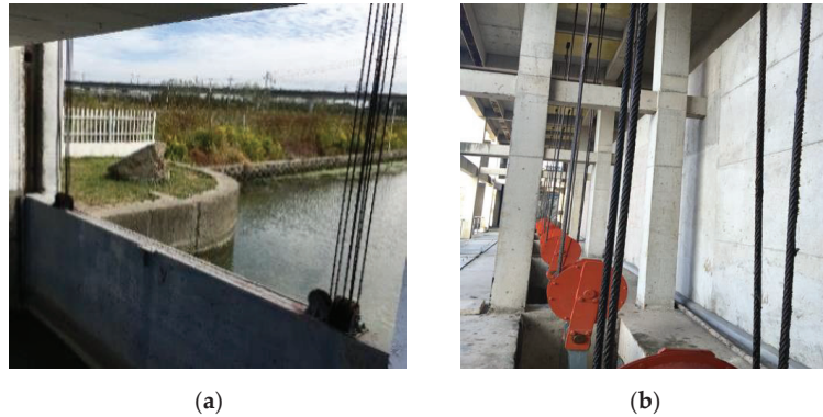
Figure 1. Sluice and wire rope working scene. (a) An example of the sluice used in rural river channels, and (b) an example of the sluice used in coastal rivers.
