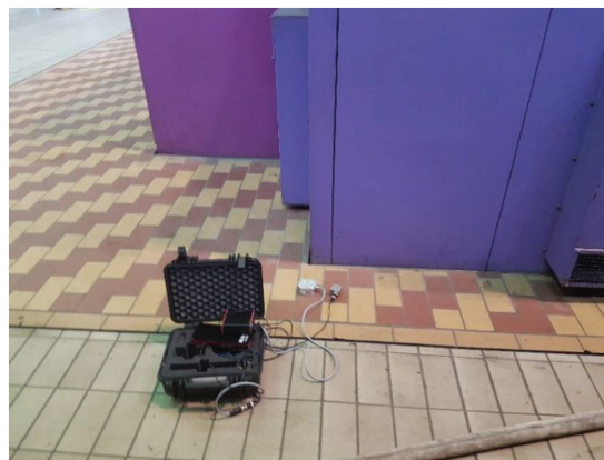
Figure 5. Measurement of vibrations at the operating speed of the turbine placed on the top plate of the foundation using a piezoelectric accelerometer.
