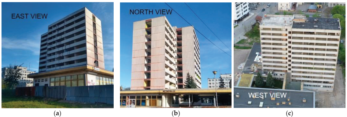
Figure 1. Examined large-panel building: (a) east side; (b) north side; (c) west side.
