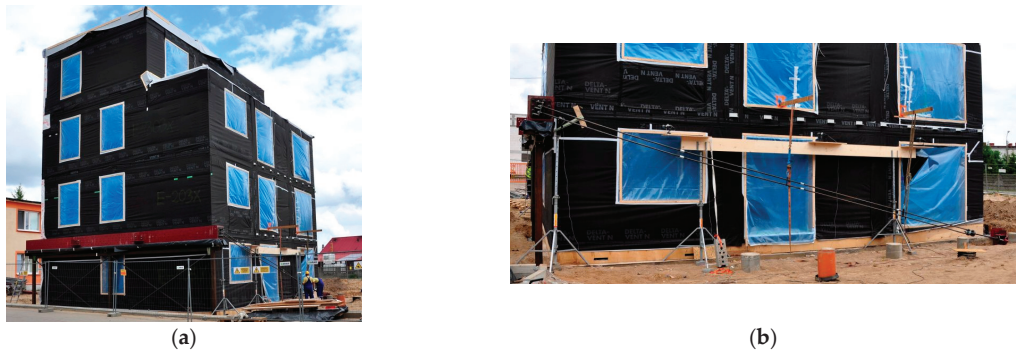
Figure 9. View of the tested building and the load application system [Fot. Unihouse SA]: (a) upper beam, traverse and (b) tie rods.
