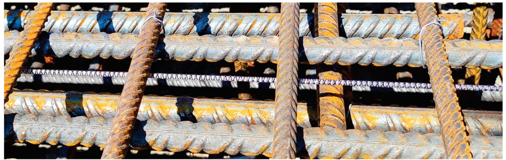
Figure 17. Installation of the monolithic sensor by tying to the existing reinforcement.
