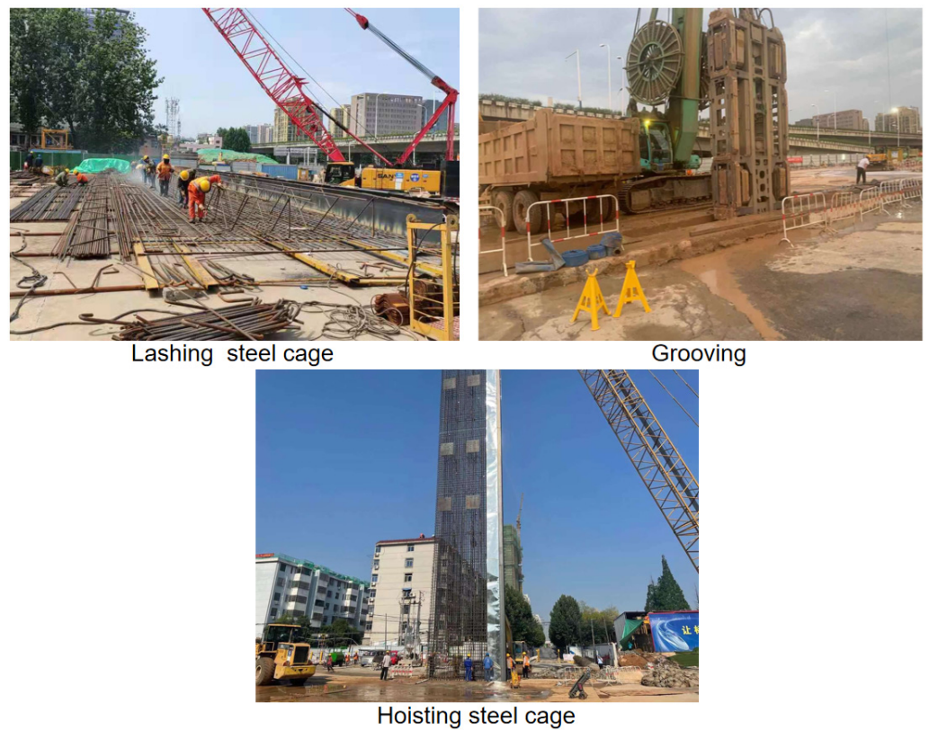
Figure 5. Construction picture of underground diaphragm wall.
