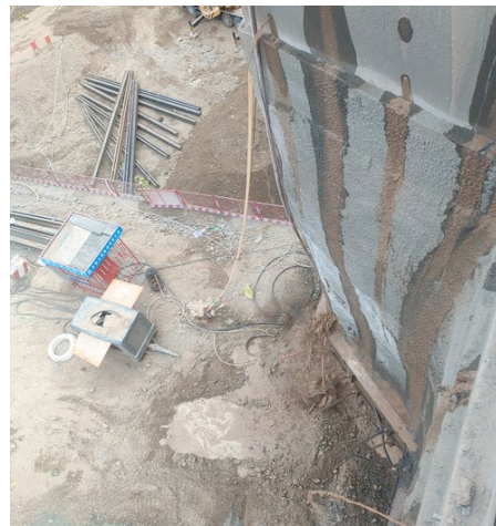
Figure 18. Pit site conditions.
