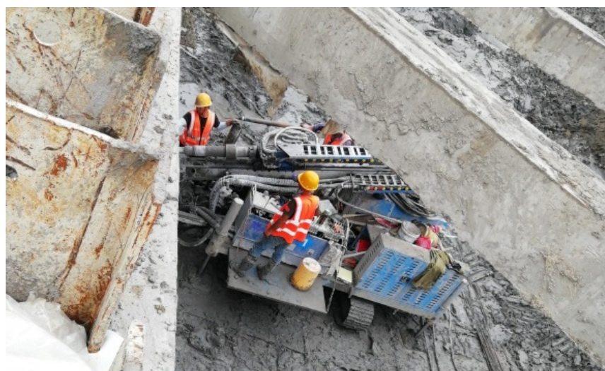
Figure 6. Grouting of anchor cables.
