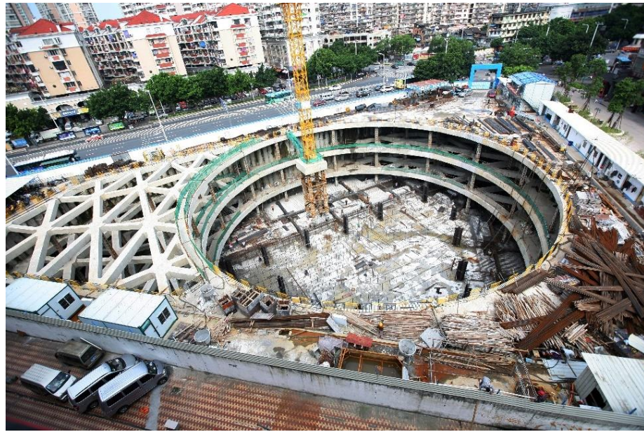
Figure 2. An image of the surrounding area of the foundation pit.
