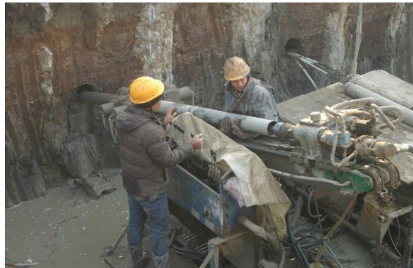
Figure 3. Drilling construction of anchor cable.
