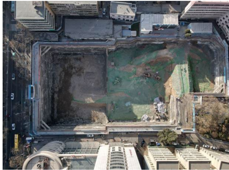
Figure 1. Map of the surrounding environment of the foundation pit.
