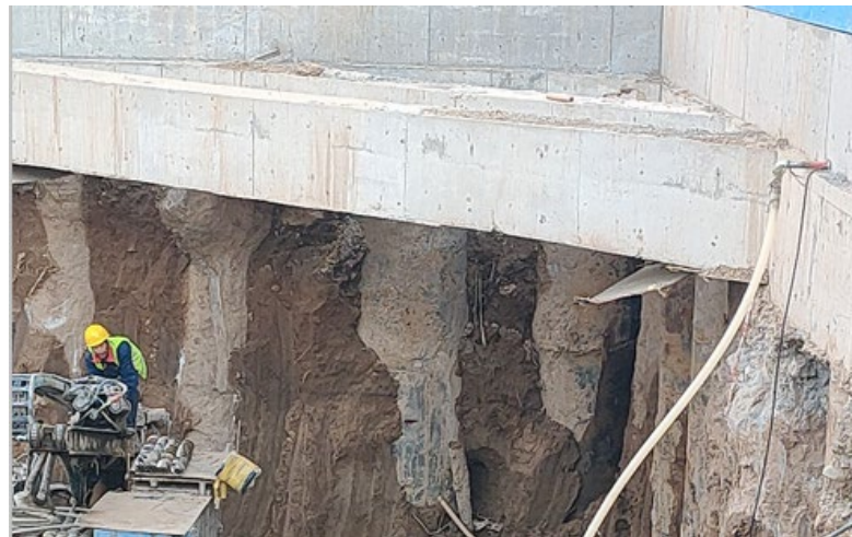
Figure 4. On-site construction of corner braces.
