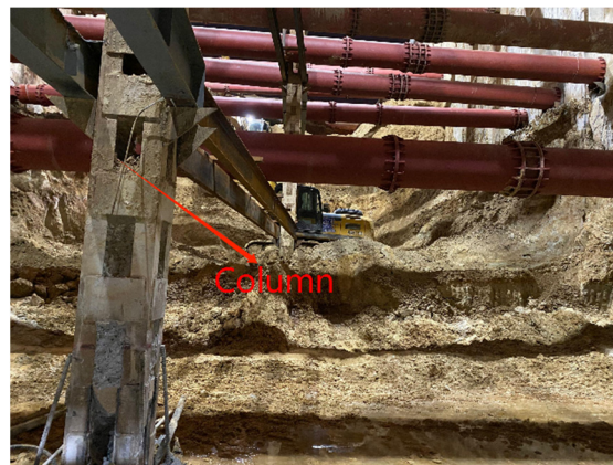
Figure 17. The construction picture of the column.
