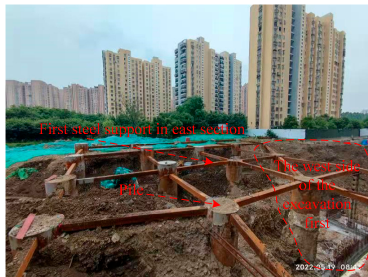
Figure 4. Foundation pit excavation site.
