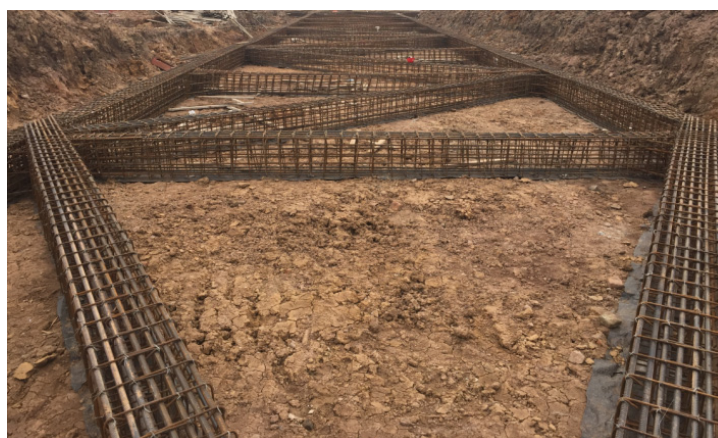
Figure 3. Steel bar binding of the inner brace.
