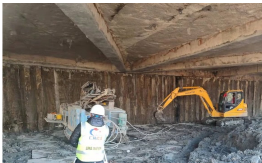
Figure 5. Drilling of the anchor cables.
