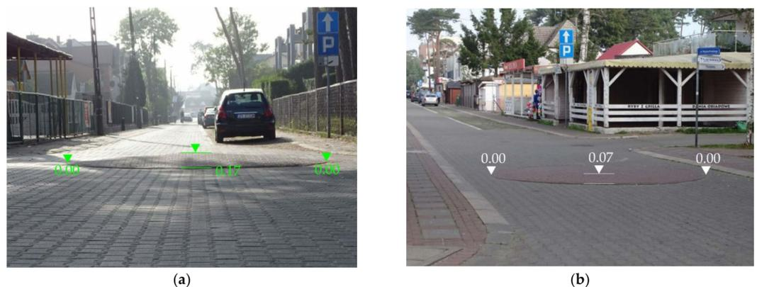
**Figure 11.** Analysed traffic circles: (a) traffic circle No. 3— $\Delta h = 0.17$  m; (b) traffic circle No. 6— $\Delta h = 0.08$  m (all dimensions in metres). Source: photo by Alicja Sołowczuk.
