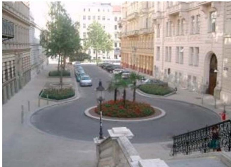
**Figure 6.** Cul-de-sac with a mini roundabout, Vienna, Austria.
