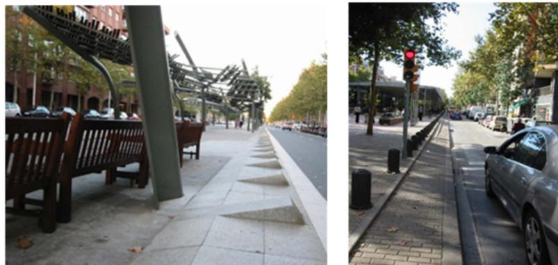
**Figure 10.** Stone elements restricting the carriageway and/or preventing illegal parking, Barcelona, Spain.
