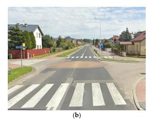
**Figure 3.** Examples of traffic circles used in Poland on two-way streets: (**a**) an example of a sectioned-off central island on a raised junction in Mierzyn, including traffic signs directing the traffic around the island. Source: photo by Alicja Sołowczuk; (**b**) example of coloured/textured surface used on the central island of a raised junction in Puławy. Source: Google Earth [5].
