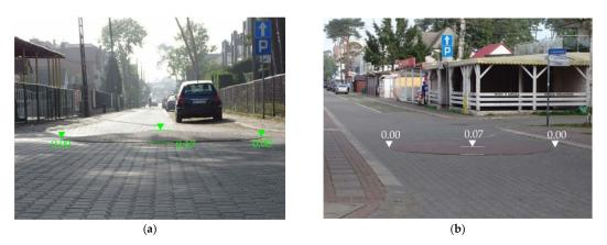
**Figure 11.** Analysed traffic circles: (a) traffic circle No.  $3-\Delta h = 0.17$  m; (b) traffic circle No.  $6-\Delta h = 0.08$  m (all dimensions in metres). Source: photo by Alicja Sołowczuk.
