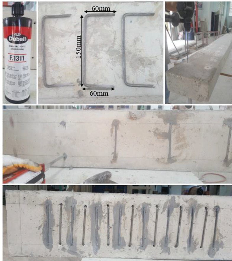
Figure 2. Strengthening beams with MSS.
