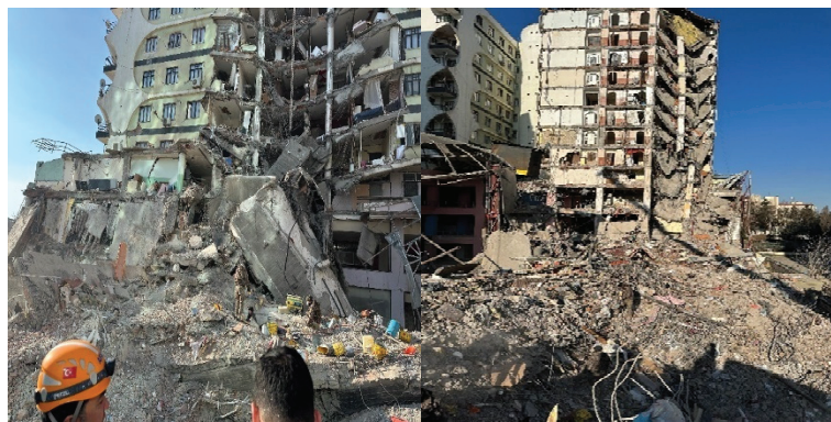
Figure 6. Collapsed buildings in Diyarbakır.
