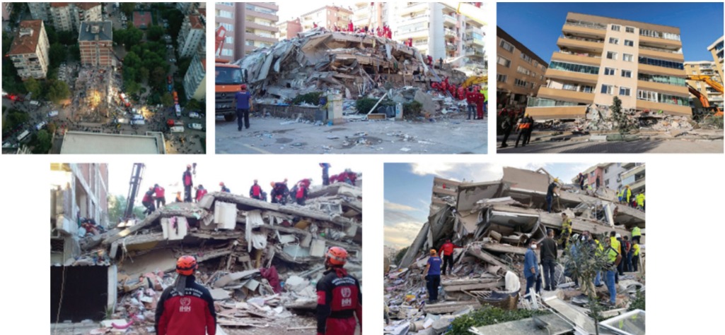
Figure 2. Images from collapsed buildings in the Bayrakli region of Izmir [28,29].
