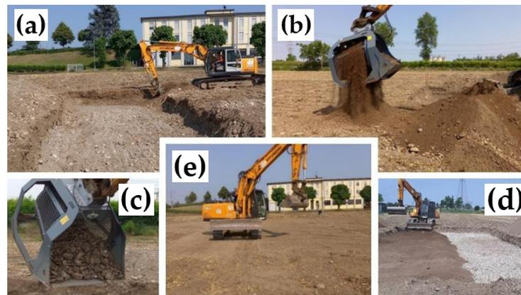
**Figure 4.** Diagram of the processing phase: (a) trenches digging; (b) soil sieving; (c) discharging of retained stones in the trenches; (d) refilling of trenches with sieved fine earth; (e) compaction of sieved fine earth layer.
