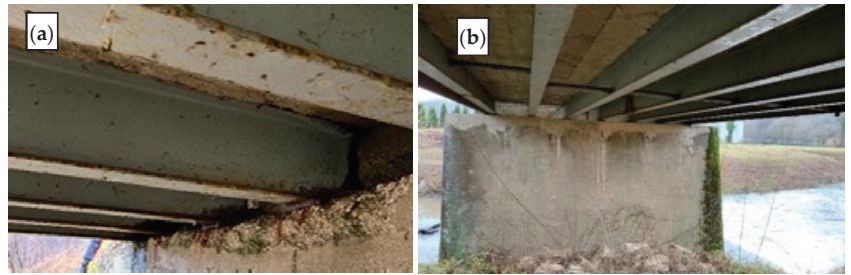
Figure 11. Svračica bridge main girder support: (a) abutment; (b) column.
