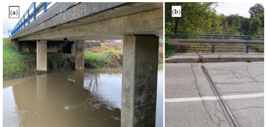
Figure 13. Prekopa bridge: (a) side view of the bridge; (b) expansion joint.
