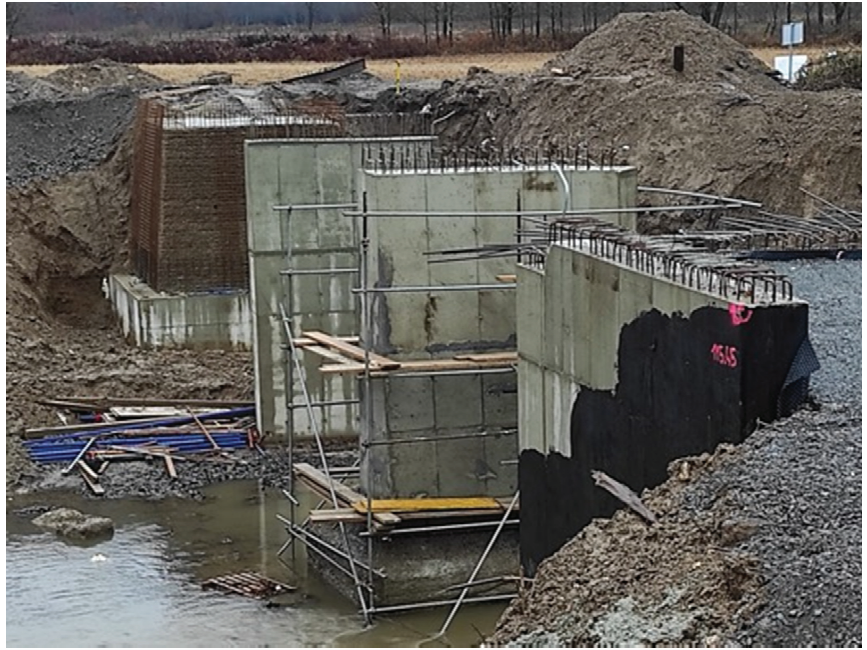
Figure 16. Progress of rehabilitation work of Matija Gubec street bridge.
