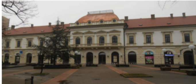
Figure 9. The Diocese in Pančevo, Serbia—a view of the front façade.
