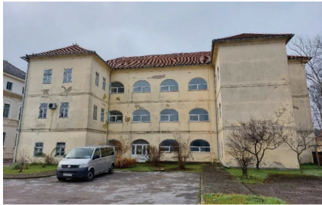
Figure 3. North-east facade of case study building.
