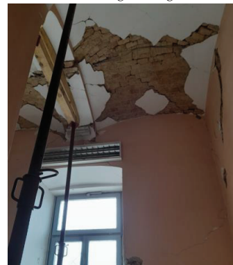
Vault damage/collapse
