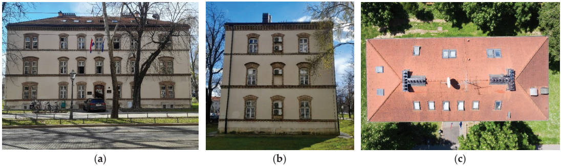
Figure 5. (a) View of the east façade; (b) View of the north façade; (c) View of the roof (photo credit: Mislav Stepinac).
