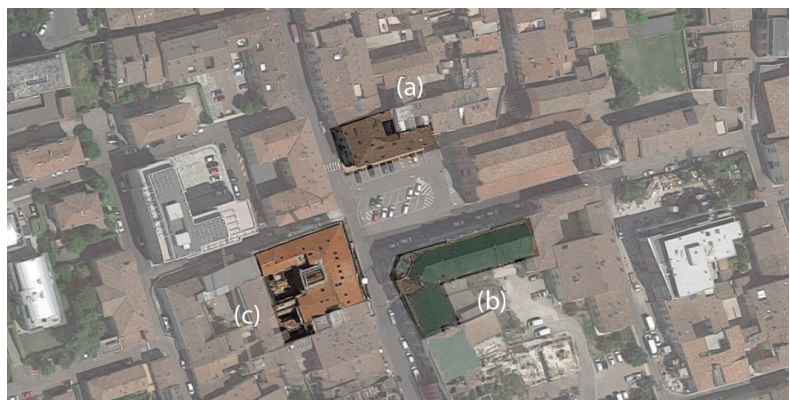
Figure 5. A view of the Mirandola case study site and the three buildings analysed.
