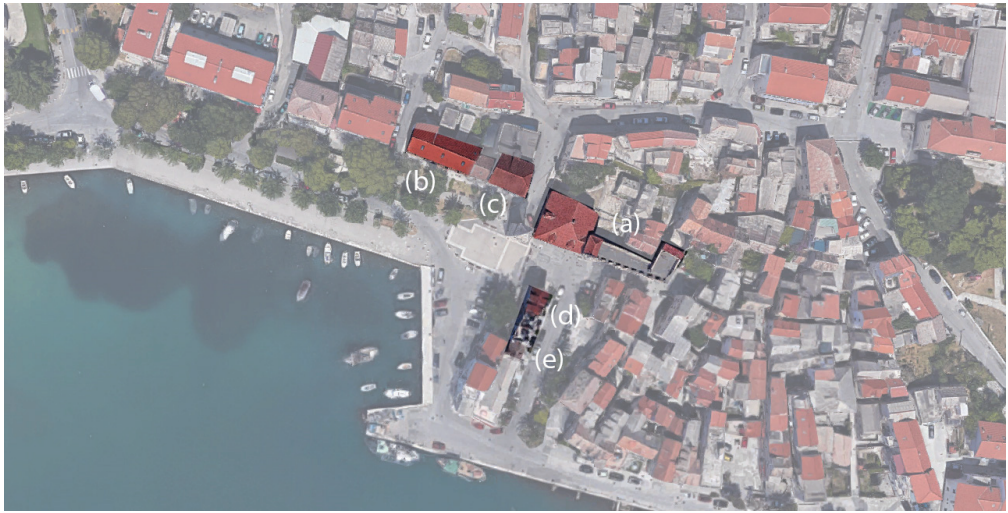
Figure 7. A view of Kaštela case study site and the five buildings analysed.
